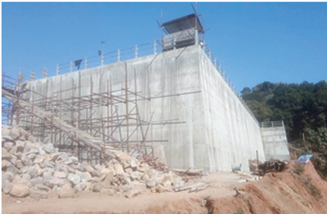
Construction of water storage reservoir located in Gopalnagar.
