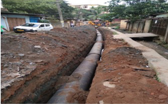
Laying of D.I pipe at North Jyoti Nagar Site
