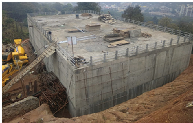
Construction of water storage reservoir located in Kenduguri.
